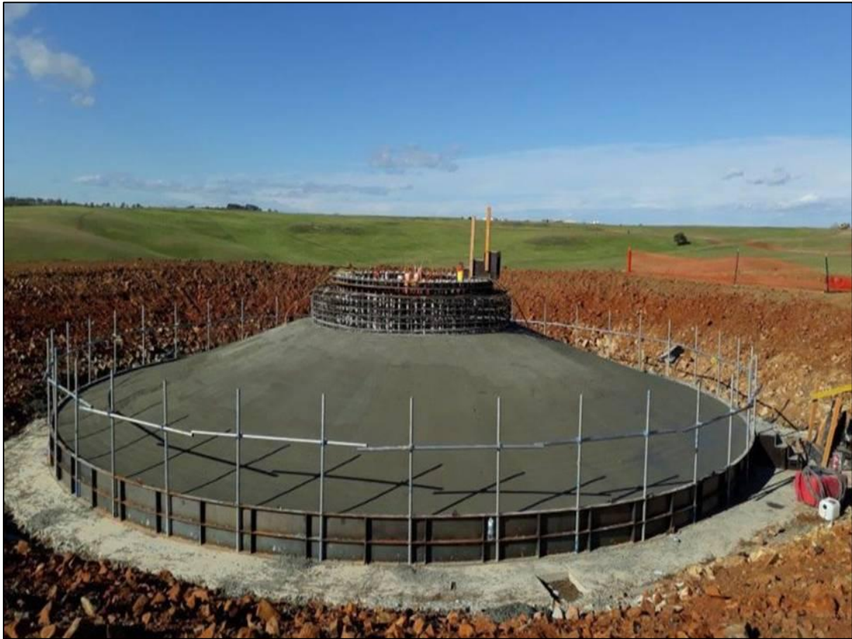
Figure 3.5: Typical Turbine Foundation
