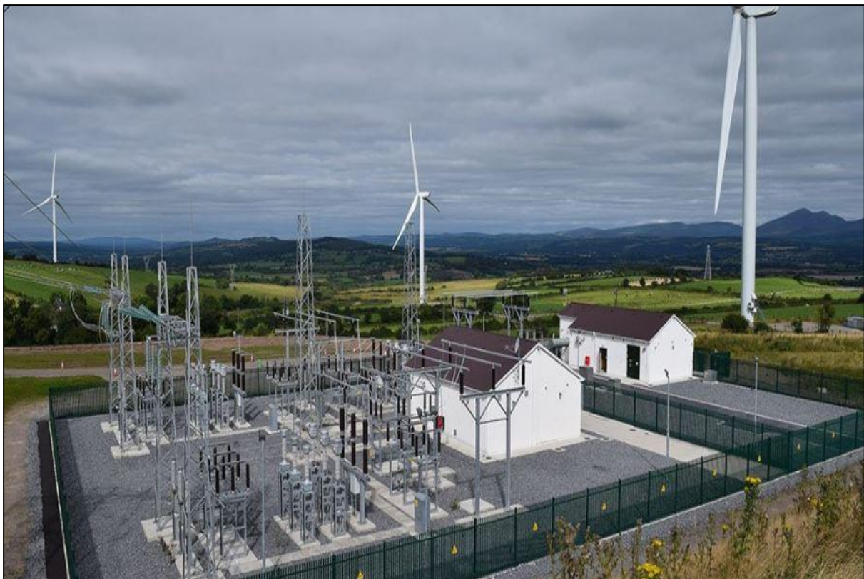
Figure 3.7: Typical 110kV substation
